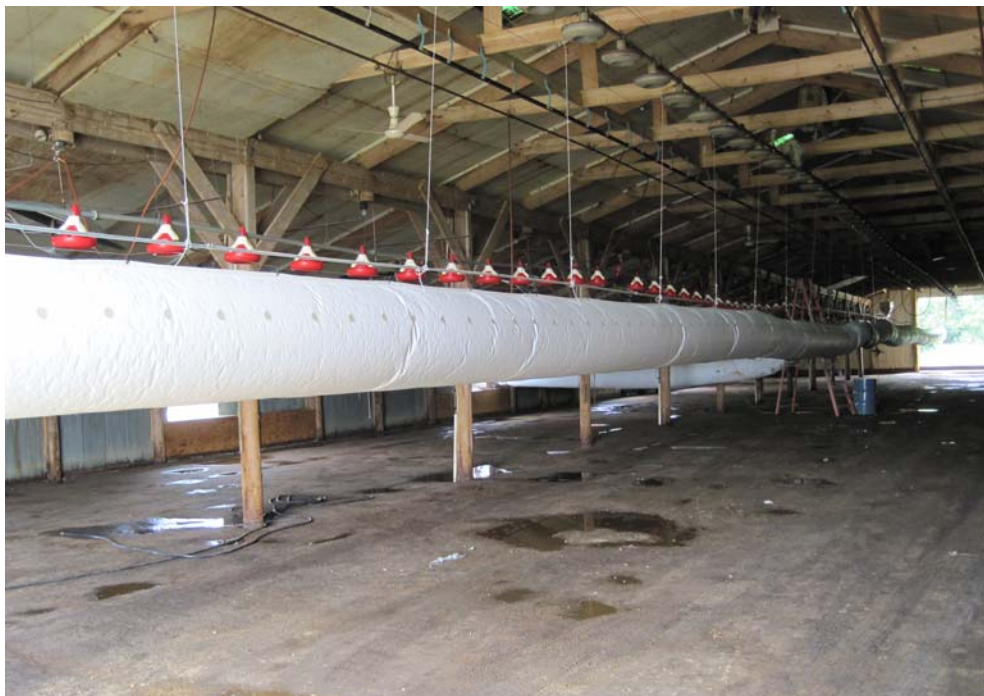
An air sock distributes the hot air inside the barn. The sock can be lowered or raised to control the temperatures at ground level.
